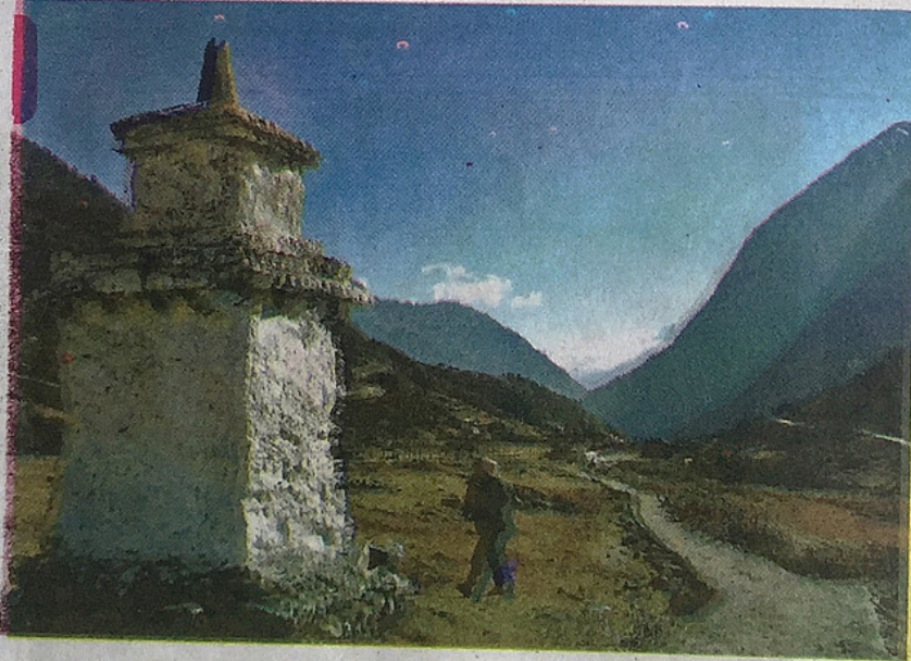
Below: An unnecessary, visually dominating cement-foot-path on flat terrain in the beautiful valley of Lachen.
